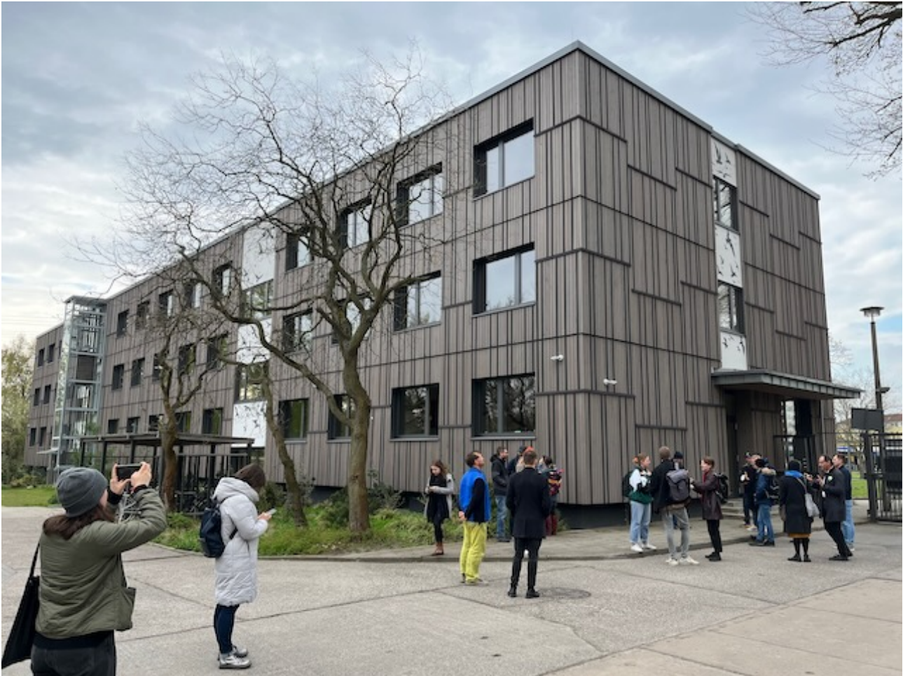
Picture 5 - Prefabricated cladding of the Berlin Zoo office building, reconstruction of a panel building from the 1960s
