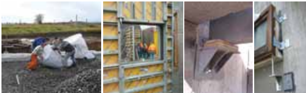
Image 1-4 Construction without thermal bridges is essential in a concrete house.
