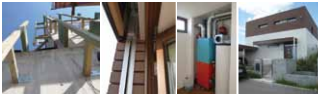
Image 5-8 Details of construction and shading, HVAC in a niche, street view (north-east) of the house.
